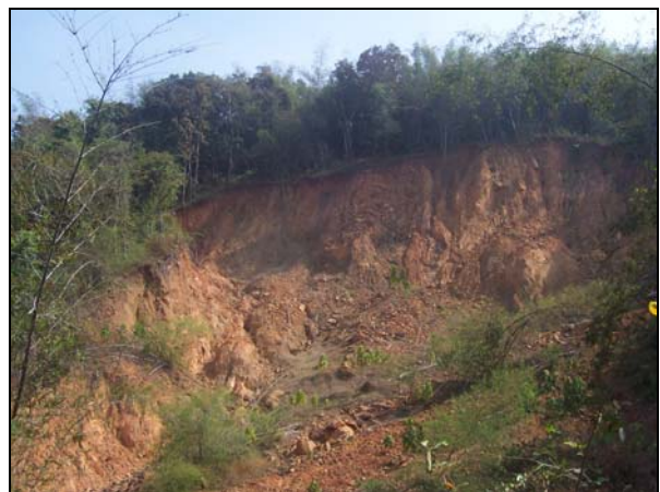
Photo 6: Crown portion showing distinct scarp of Neriya debris flow.
