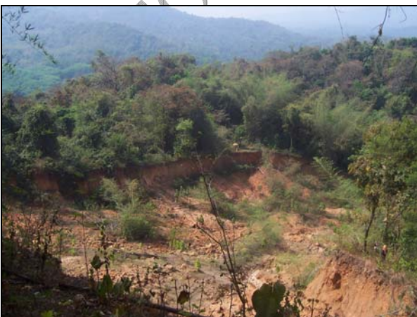
Photo 5: Down stream view of present day Neriya debris flow from the crown portion.
