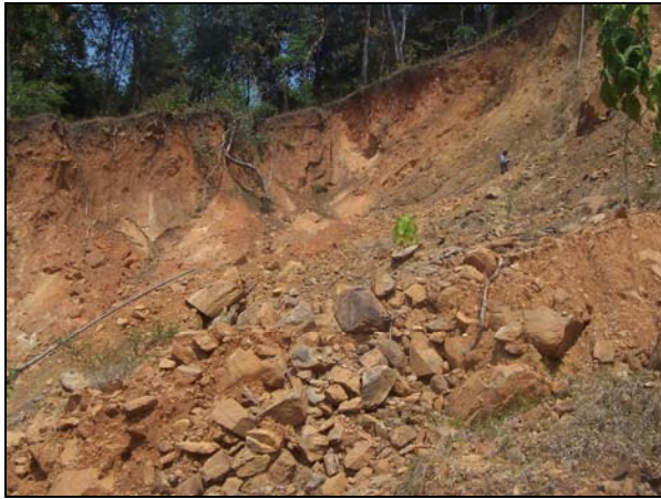
Photo 7: Dislodged blocks of dyke rock exposure just below crown portion
