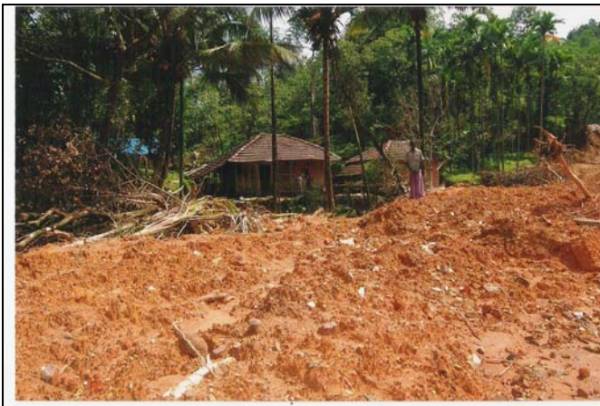
Photo 3: The heaped up debris material at toe part day after slide on 14.08.08. (Photo courtesy Village Panchayat Neriya)
